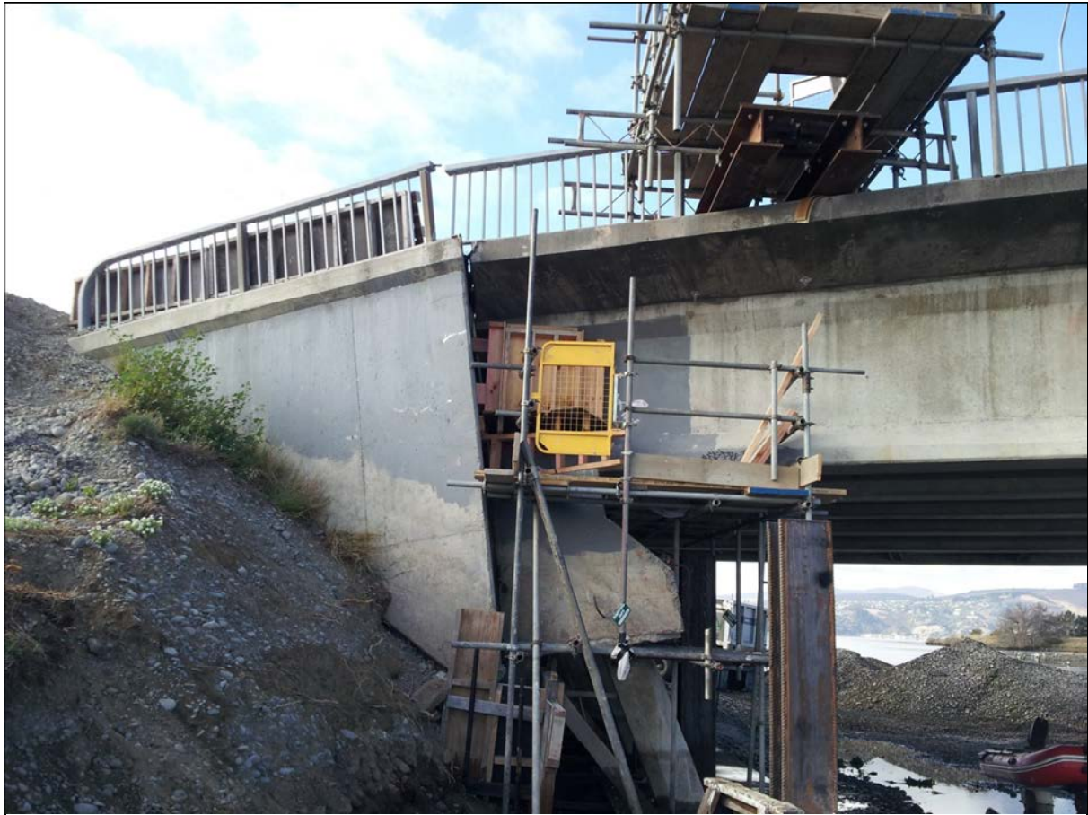
Figure 5: Rotated western abutment and temporary pile for abutment.
