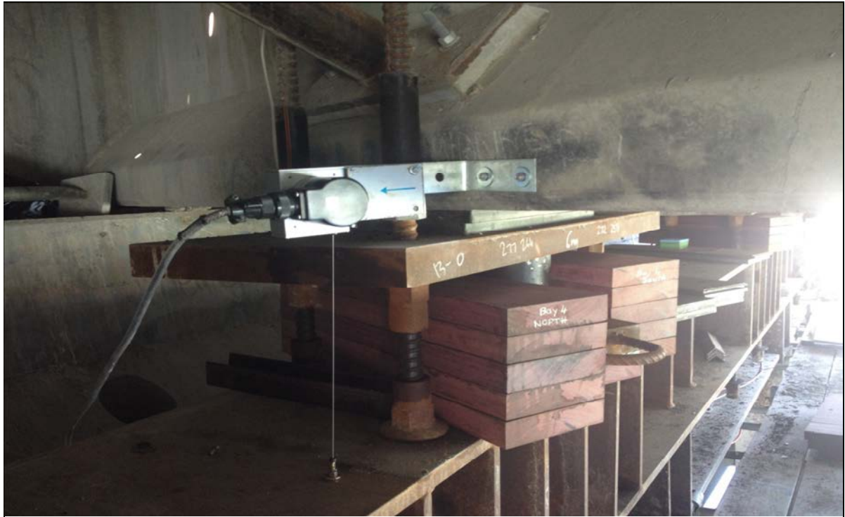
Figure 17: Jacking and Packing on Temporary Abutment
