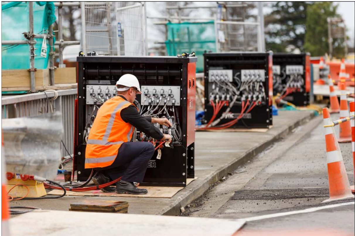
Figure 12: Linked Synchronous Lifting System Pumps placed across the Bridge
