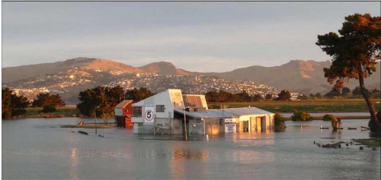
Figure 3: Pleasant Point Yacht Club after the Earthquake
